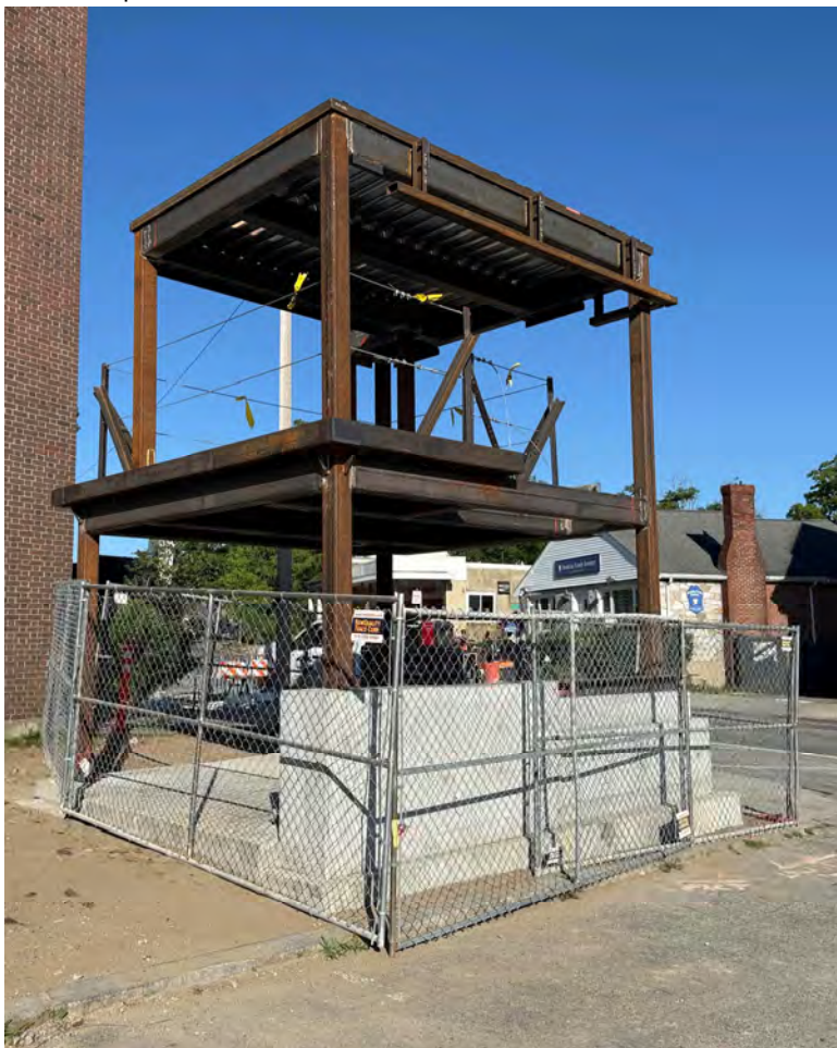
Mock-up with steel frame and deck.
